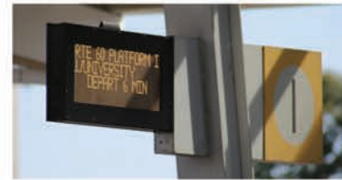
Installed digital signs at DART Central Station to display real-time information and allow riders who are blind to hear information.
